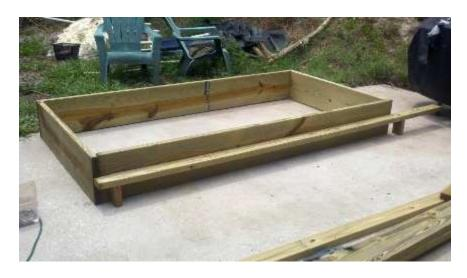
First, notice that the 2X4 is on-edge, and has one end flush with the end of the structure, not simply flush with end of the 2X12 on that side. The other end extends past the structure. Also note the two spacers the 2X4 sits on. Once the height was determined, half way up the side, those two spacers were cut to the exact same size. These will be used for the remaining sides, as well as any other ponds to be built. So long as the pad the pond sits on is
