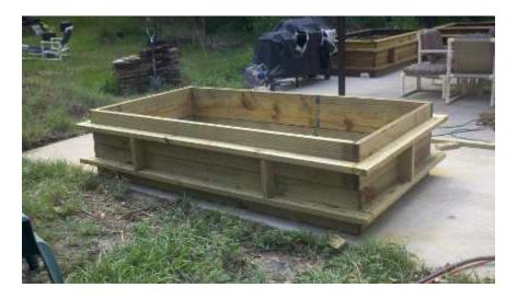
Here is where you decide where to put the over-flow fitting. I placed mine about a foot from the corner, more-or-less, as close to the top as I could, while still allowing for the cap rail to sit on top of the frame. The fitting has a thickness of plastic that must be allowed for, or be trimmed at the top once in place, so that it does NOT stick up above the frame. This does mean that the water level will never be any higher than the bottom of that fitting. Just something to keep in mind.
