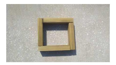
I use 5 of the 3in. deck screws in each joint. Note that one end of each board is covered, the other end exposed. It is important that the above pictured pattern is followed, to maintain the shape and structural integrity.
