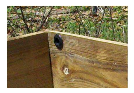
The top of that fitting is just low enough so it clears the liner. Of course, this picture was taken before the line was fitted, otherwise, the black-on-black would have been hard to see.
