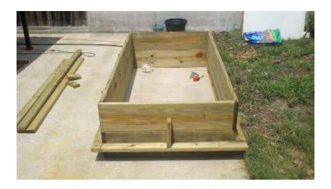
If you are using just a single spacer on the ends, as I did, don't finish screwing the frames to those vertical spacers, just yet. Use the remaining 2X4's to make the upper rails, starting with the long sides, screw them in place from the inside, using the tape measure to mark the screw points just like you did for the lower rails. Once done, add the two end rails, making sure the piece sits down on the spacer, and that both ends are even with the side rails.
