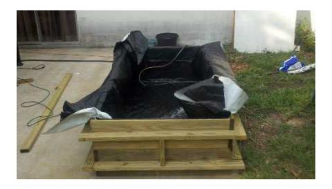
Make sure the liner goes all the way to the bottom where the wood frame meets the base. You do not want any space at the bottom where there is any gap between liner and wood. Start adding water so there's only about of inch of water, then you should be able to pull gently up from the sides, to minimize any wrinkles on the bottom. Note I said "minimize." It would seem that perfection is seldom attained! Just go for what you can live with, but do the best you can.
