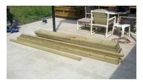
Take two of the 2X12's and cut them exactly in half. These four pieces will become the short sides of the two levels. Two show how the 2X12's are laid out and fastened, here's the basic idea demonstrated with some scrap 2X4's, in the next picture. I guess you could call it a "basket weave" pattern.
