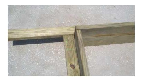
Here is where that carpenter's triangle would come in handy. I used it to draw a line to cut off the extended ends at each corner. (Not that green line
